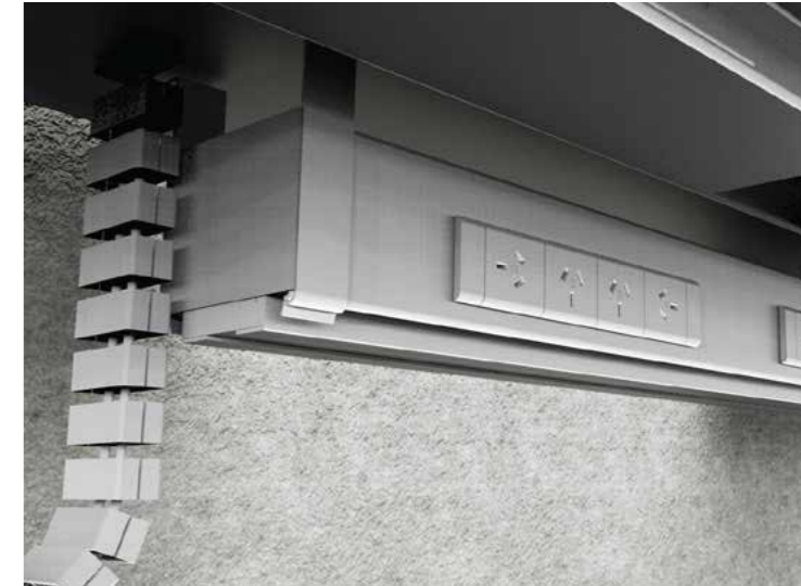
SUBWAY CABLE TRAY (UNDER)
